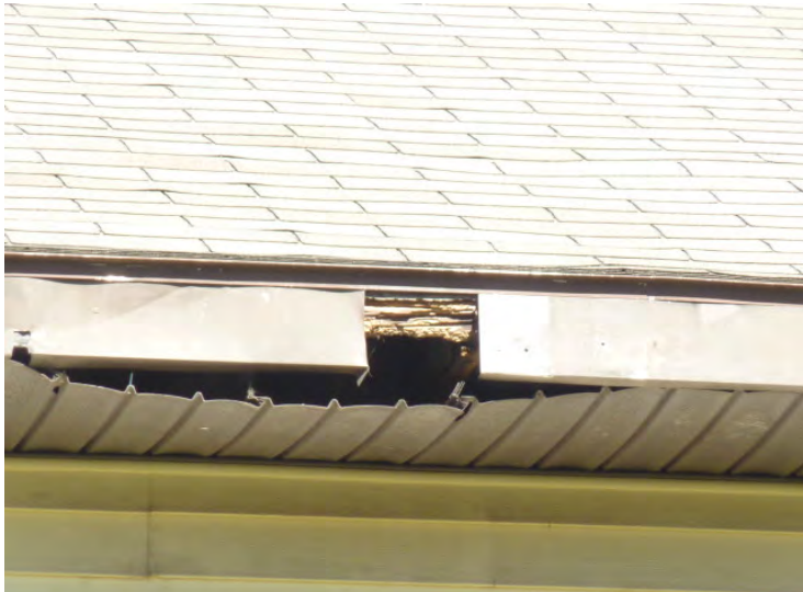
Typical site-wide fascia and vinyl siding/soffit failures.
