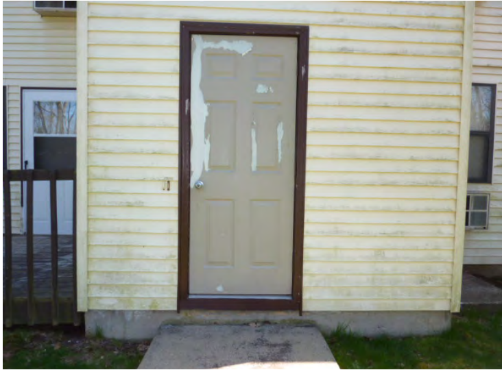
Exterior steel building entrance and egress doors are the originals and are scheduled to be replaced early in the term.
