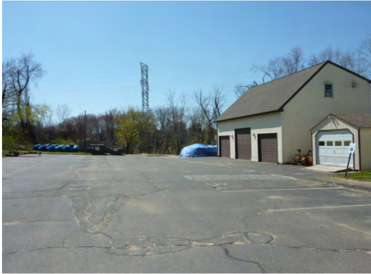
Asphalt paving at service garages and trash yard has significant historic crack sealing, new cracking, and sub-base failures property-wide.
