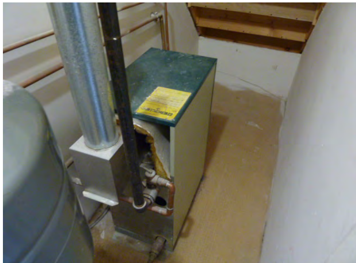
Gas-fired heating hot water boiler beneath stair (shown at top of picture) in 2-story 2-bedroom apartments is required to be in a fire-rated room in Year 1.
