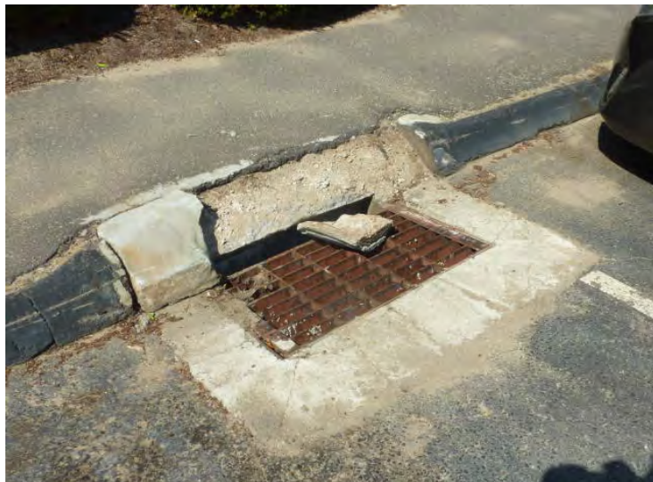
Premature failure of concrete catch basins and curbs require their total replacement early in the plan.
