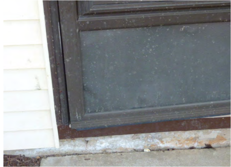
Typical twisted storm door does not close properly and is shown to be replaced.
