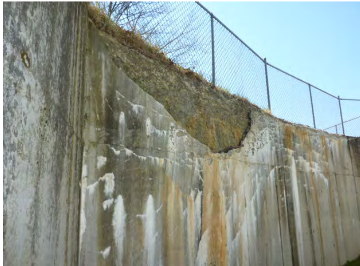
Finish on concrete retaining wall is stained and failing.
