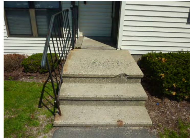
Typical trip hazard (risers of varying heights and misaligned concrete paving slabs) at concrete stoops should be eliminated and new rails provided.
