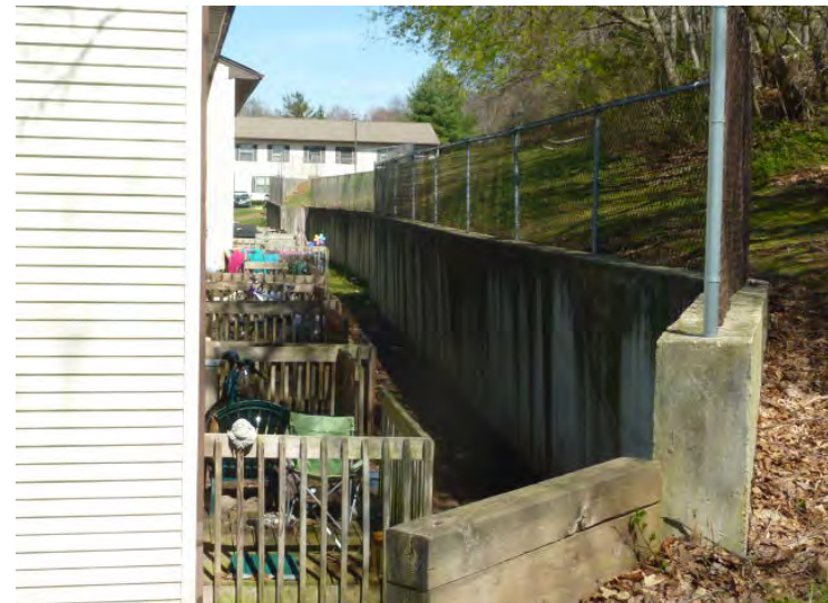
Retaining wall and chain link fence require repair. Wood decks behind Building 2 and ramps behind accessible units at Buildings 2, 3, and 5 require repairs and paint.
